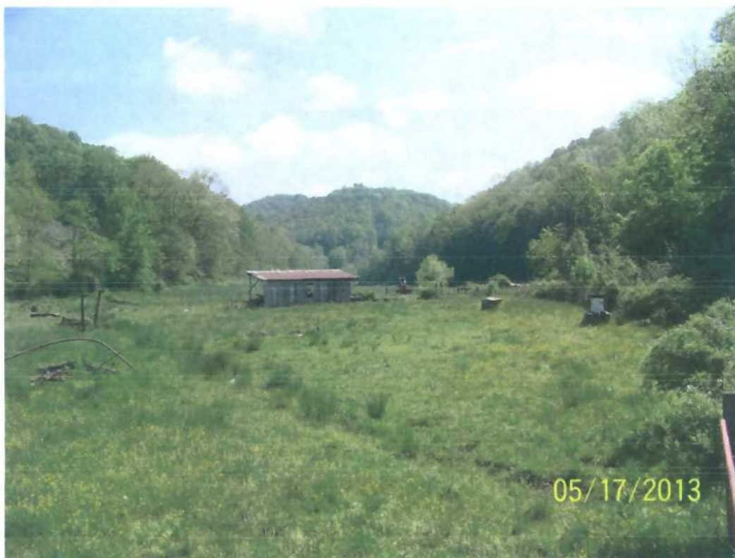
Figure 3.4 Floodplain area looking East
