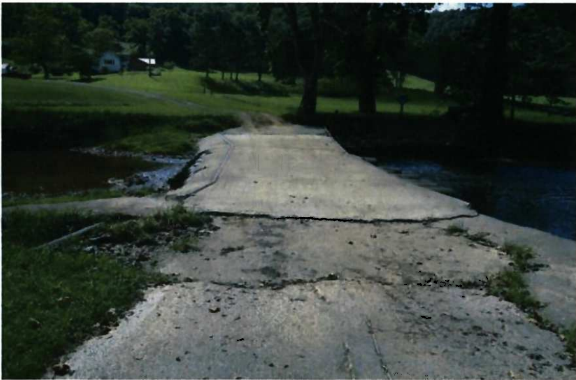
Photo #2: View west across Stream 1 (second crossing at existing access road/bridge)
