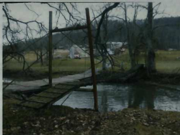
Footbridge to Gessler Property Facing West
