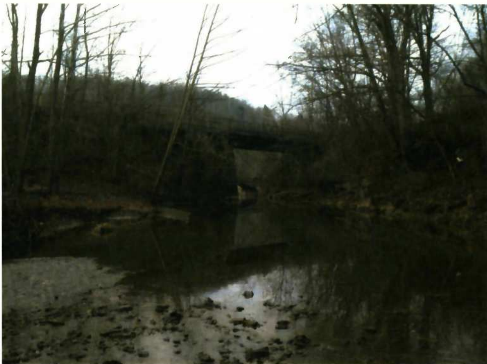
Figure 3.4 Arnolds Creek looking south (typical stream section & RR bridge)
