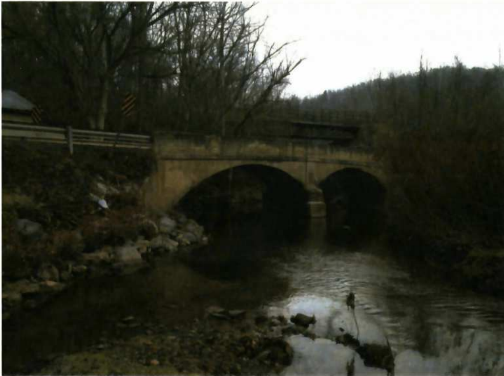
Figure 3.3 Arnolds Creek looking north (typical stream section & CR bridge)
