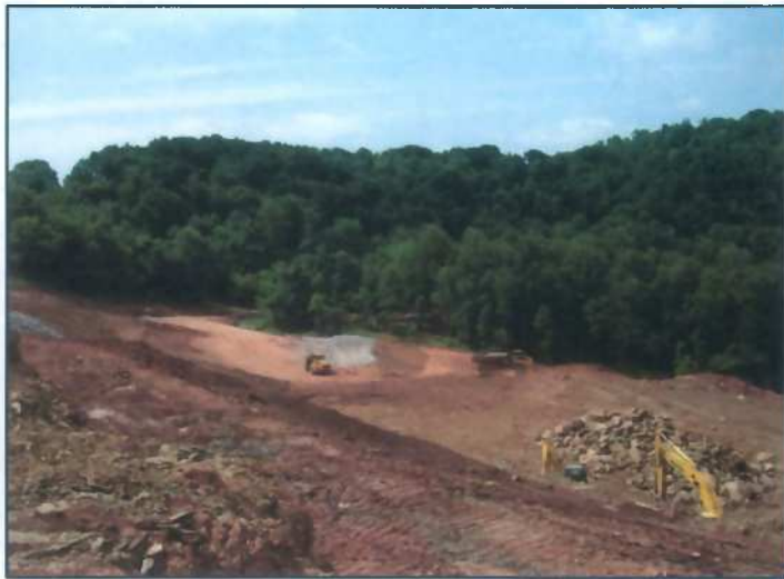
3) Proposed John North Well Pad – under construction
