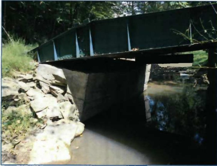
5) Left buttress facing downstream
