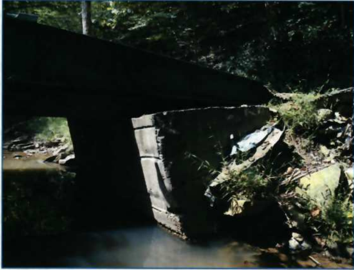
9) Right buttress facing upstream
