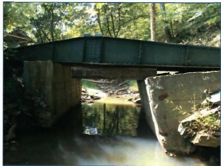
8) Nazareth Farm Bridge facing upstream
