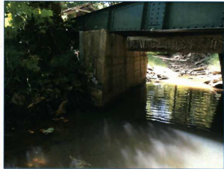
10) Left buttress facing upstream
