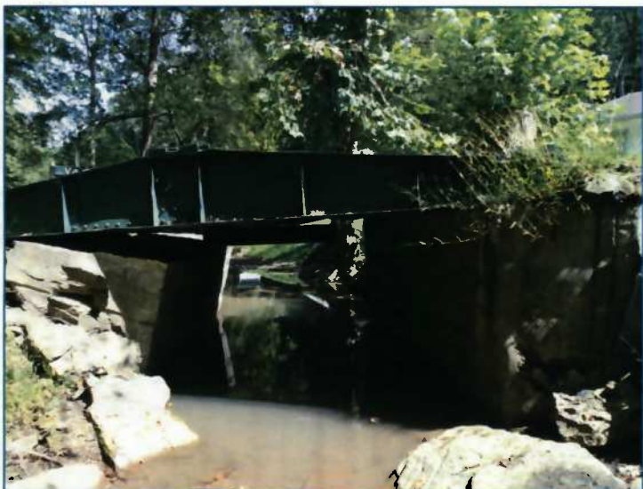
3) Nazareth Farm Bridge facing downstream
