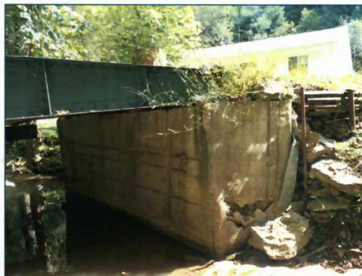
4) Right buttress facing downstream
