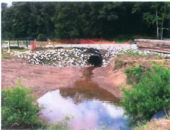
Existing Culvert (Upstream)
