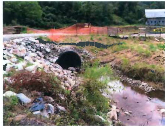
Existing Culvert (Downstream)
