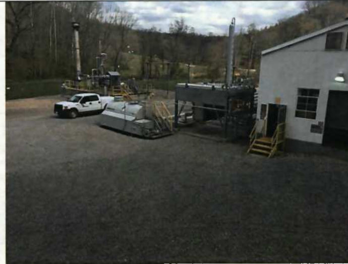
Photo: 4 Date: 4-28-2015 Comments: View of existing compressor building, and location of proposed new building, facing east.
