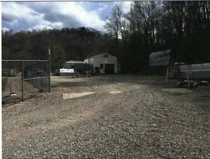
Photo: 1 Date: 4-28-2015 Comments: View of the existing gravel access drive and lot associated with the Maxwell Compressor Station, facing south.
