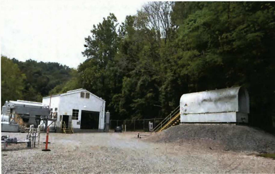
Photograph 6. Proposed Building Location (Building will Replace Existing Tank)
