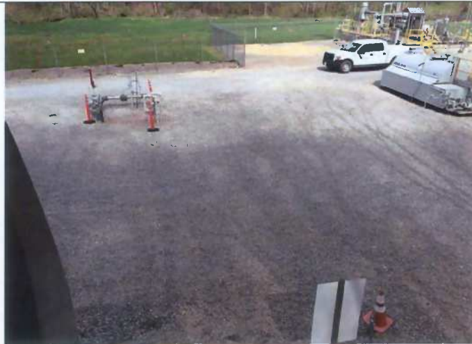
Photo: 3 Date: 4-28-2015 Comments: Overview of location of new compressor building, approximately 40 feet in front of the existing building, facing ENE.
