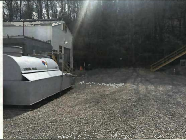
Photo: 2 Date: 4-28-2015 Comments: View of proposed workspace associated with the new building installation, facing WSW.
