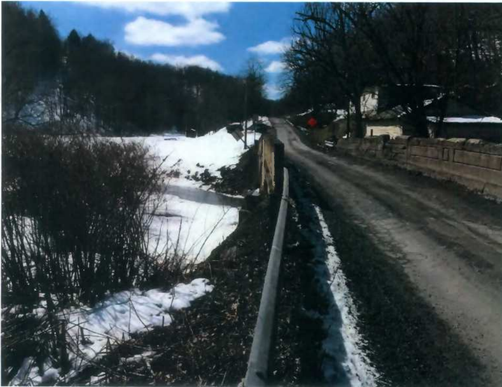
Central Station Bridge, facing west
