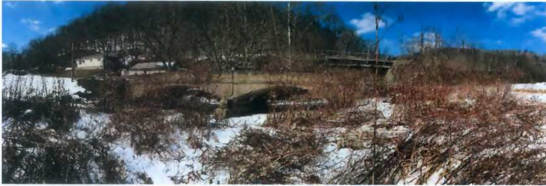
Arnold Creek, downstream view
