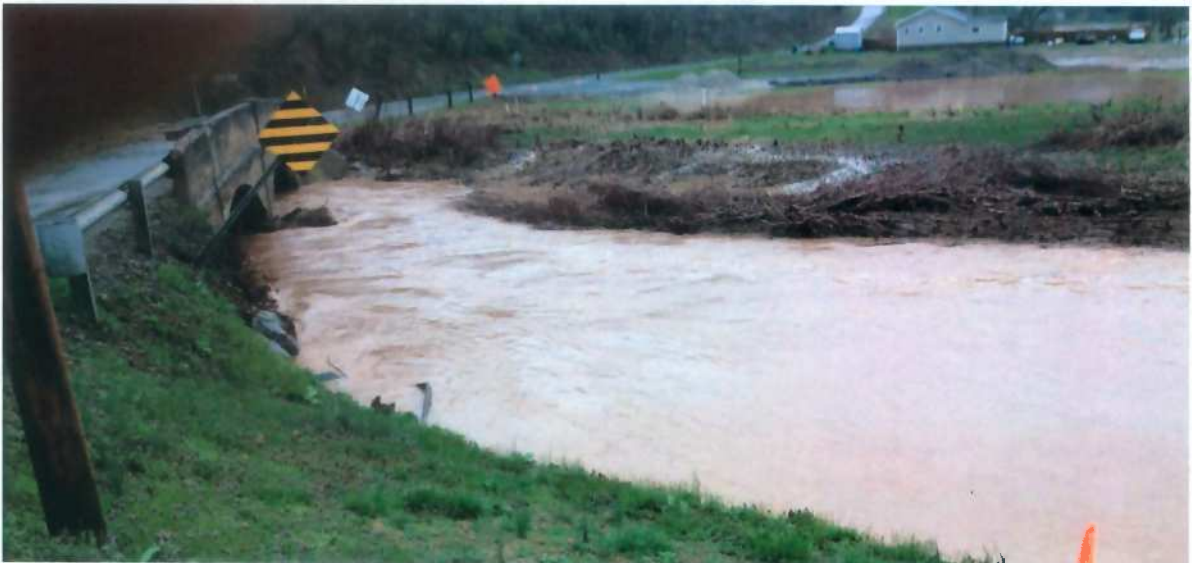
Central Station Bridge, Arnold Creek – April 10, 2015
