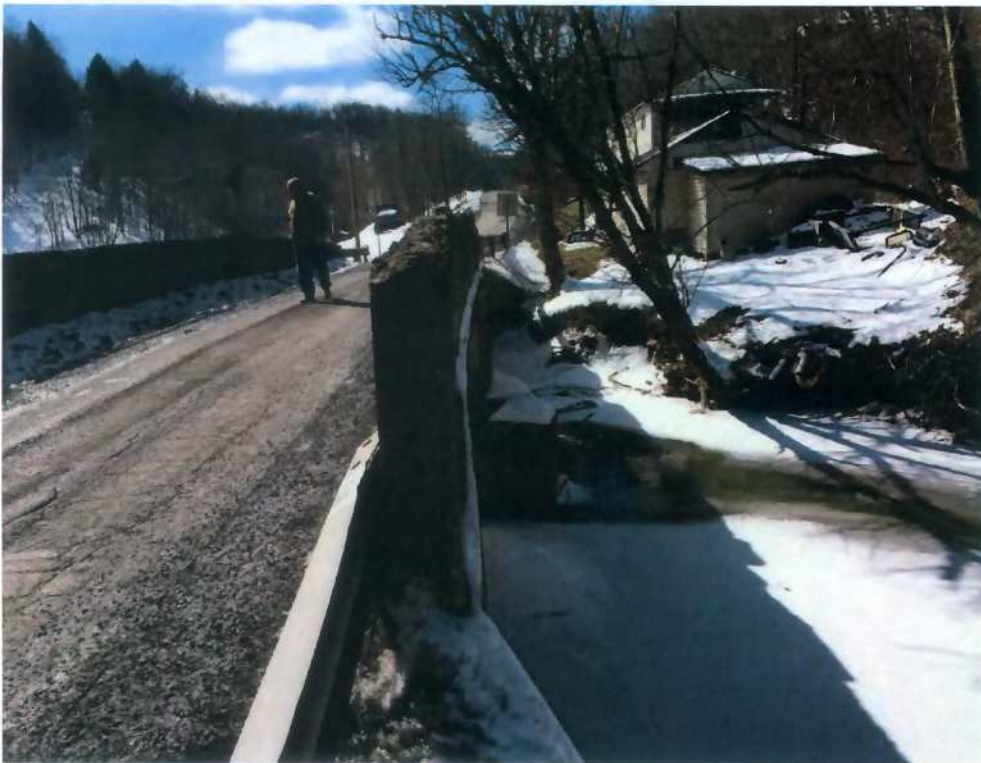
Central Station Bridge, Arnold Creek, upstream view
