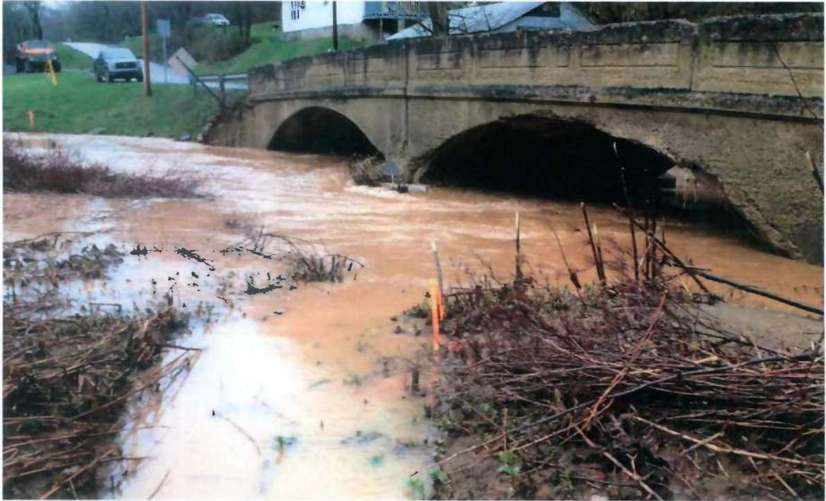
Central Station Bridge, Arnold Creek – April 10, 2015
