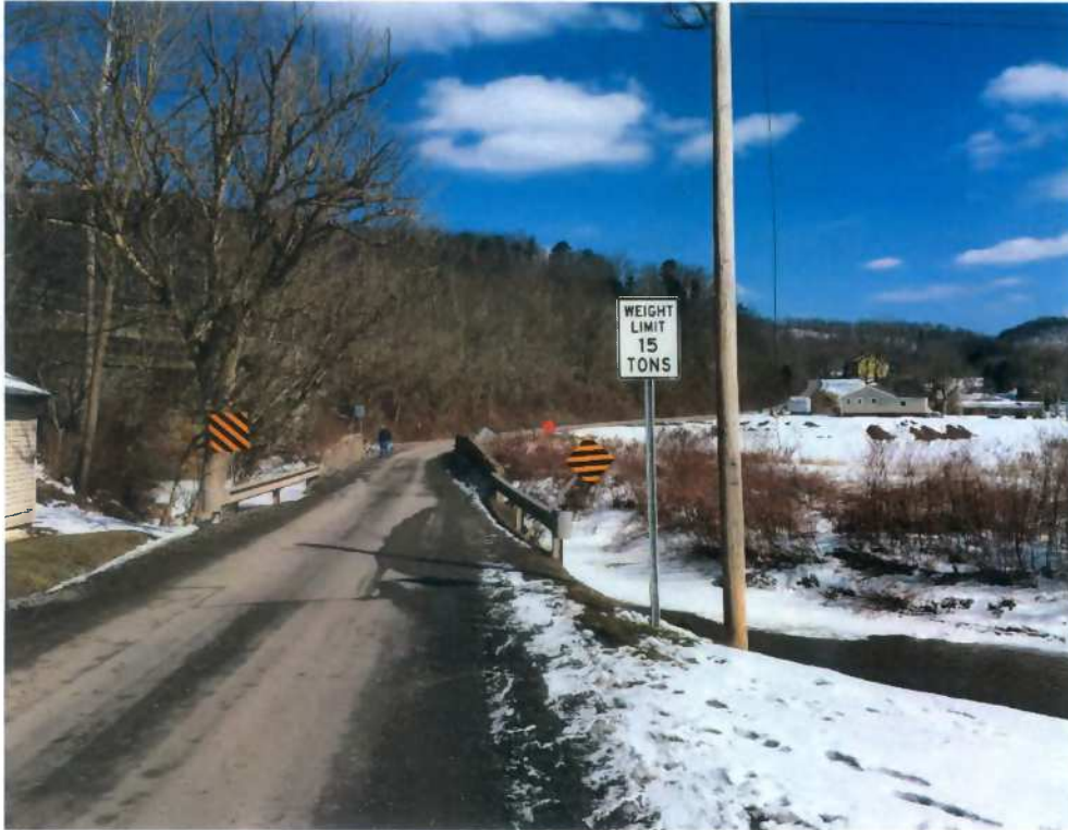
Central Station Bridge, facing east
