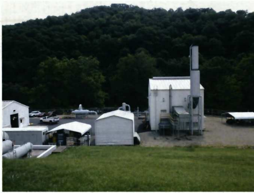
PHOTO 1 Existing compressor station.
