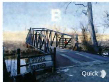
B EXISTING BRIDGE
