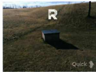
R EXISTING WELL HOUSE (PLUG & ABANDON WELL)
