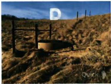
D EXISTING WATER TROUGH / DEVELOPED SPRING
