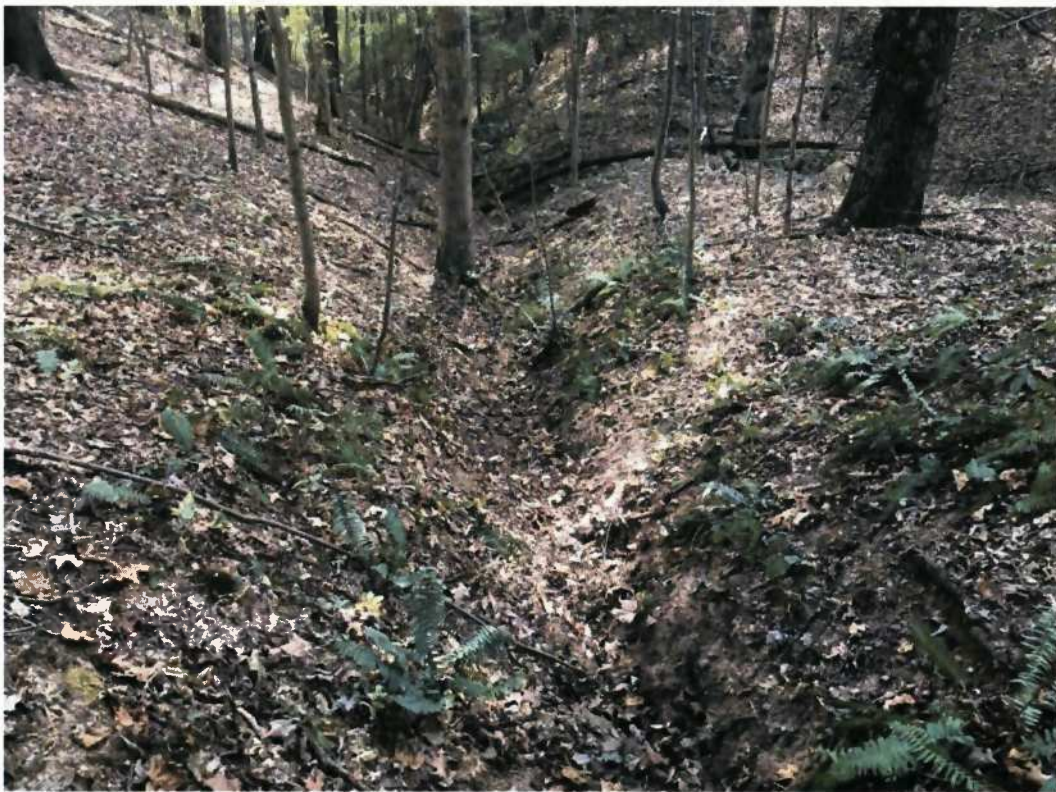
Photo 73. View of S45 facing south downstream (09/26/2016)
