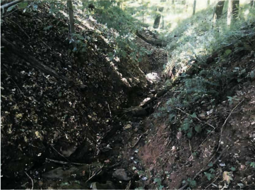
Photo 48. View of S21 facing south downstream (08/26/2016)
