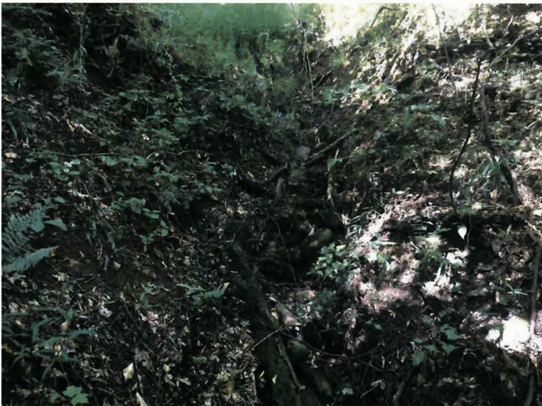
Photo 49. View of S22 facing south/southeast downstream (08/26/2016)
