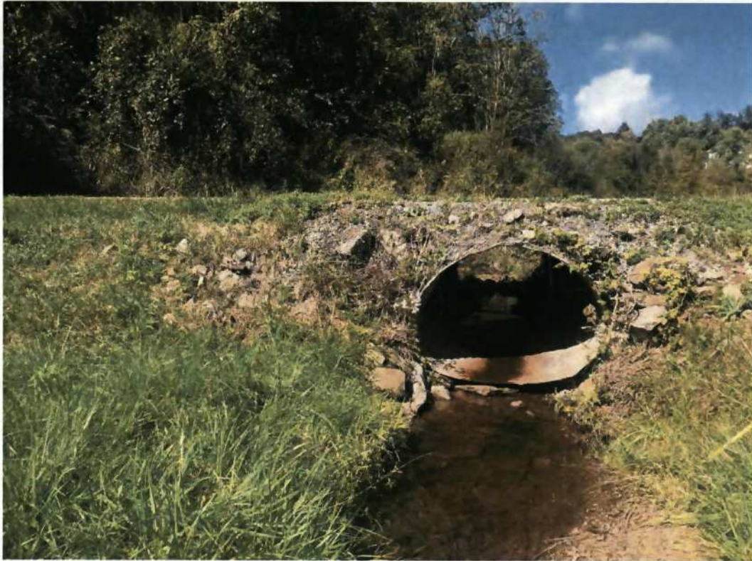
Photo 80. View of S52A at existing access road crossing facing northwest upstream (10/03/2016)
