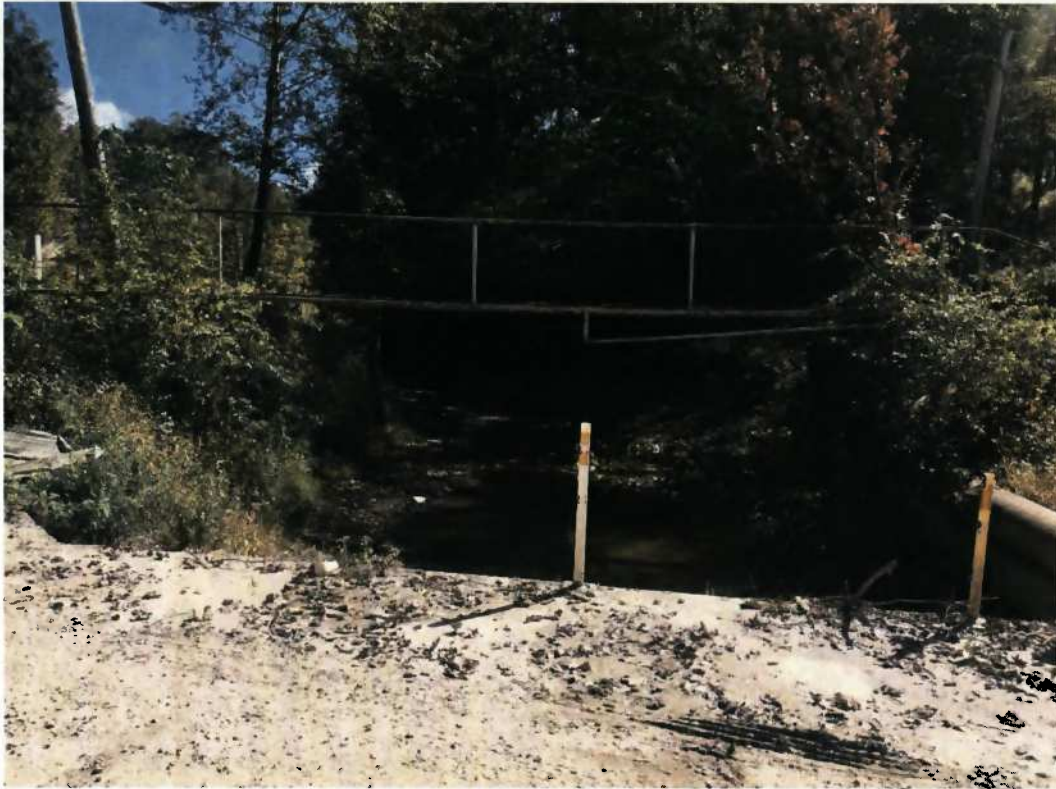
Photo 84. View of S55 at existing access road facing southeast downstream (10/03/2016)
