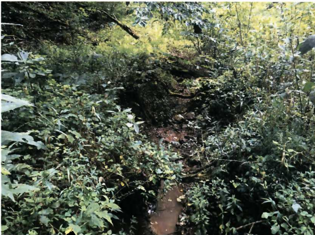
Photo 35. View of S8 facing south downstream (08/25/2016)
