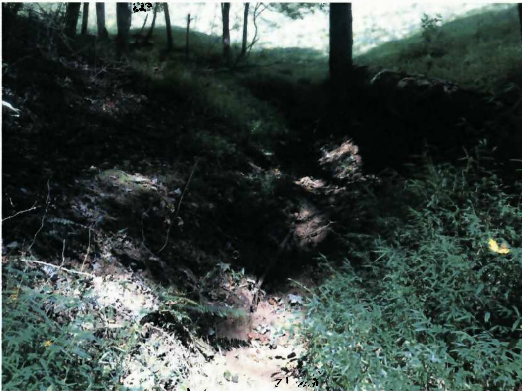
Photo 47. View of S20 facing north/northwest upstream (08/26/2016)
