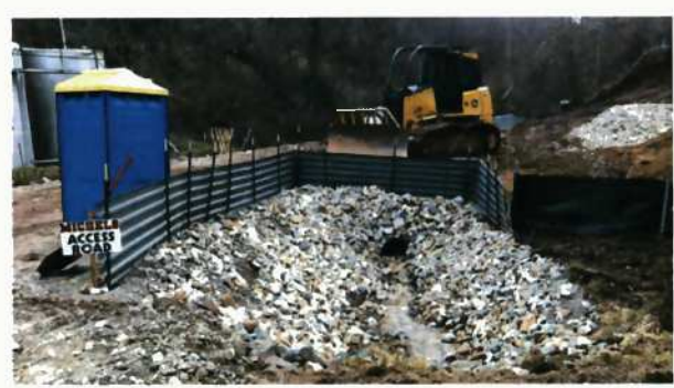
37C SUPPLEMENTAL 404 CWA BMP CONTROLS NTS DETAIL PROVIDED BY ANTERO MIDSTREAM LLC
