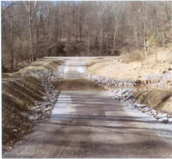
Existing Ford Facing East
