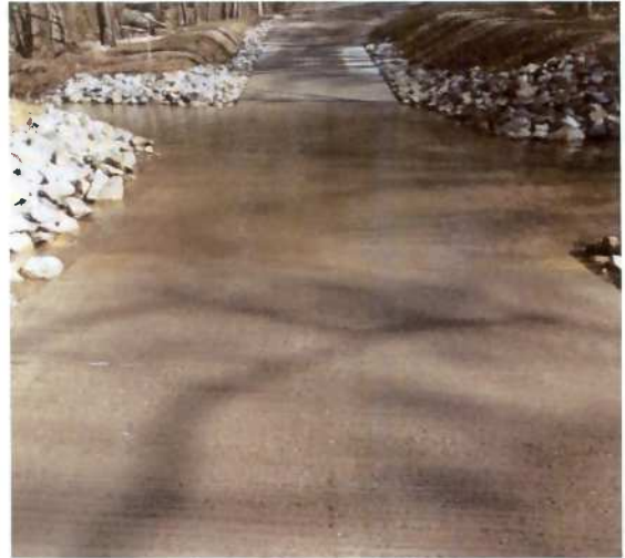
Existing Ford Facing West
