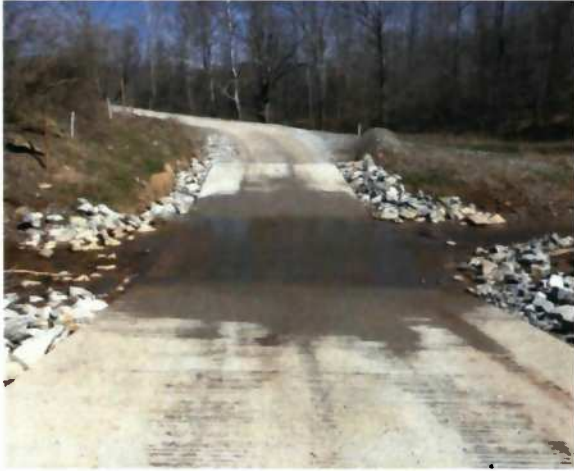
Existing Concrete Ford
