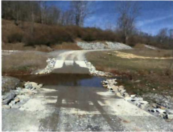
Existing Concrete Ford
