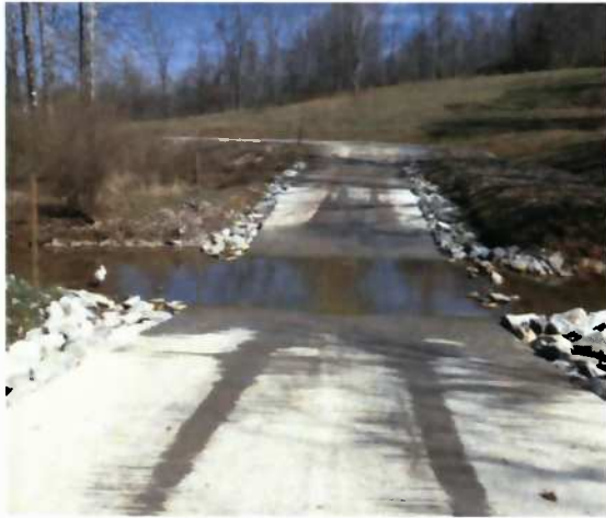
Existing Concrete Ford
