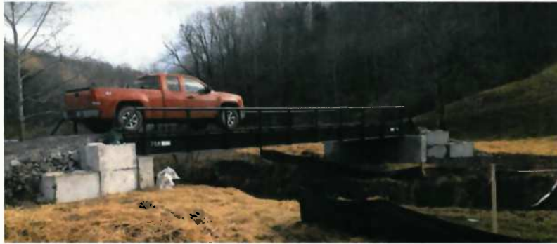
Example Bridge (Similar to Proposed Bridge)
