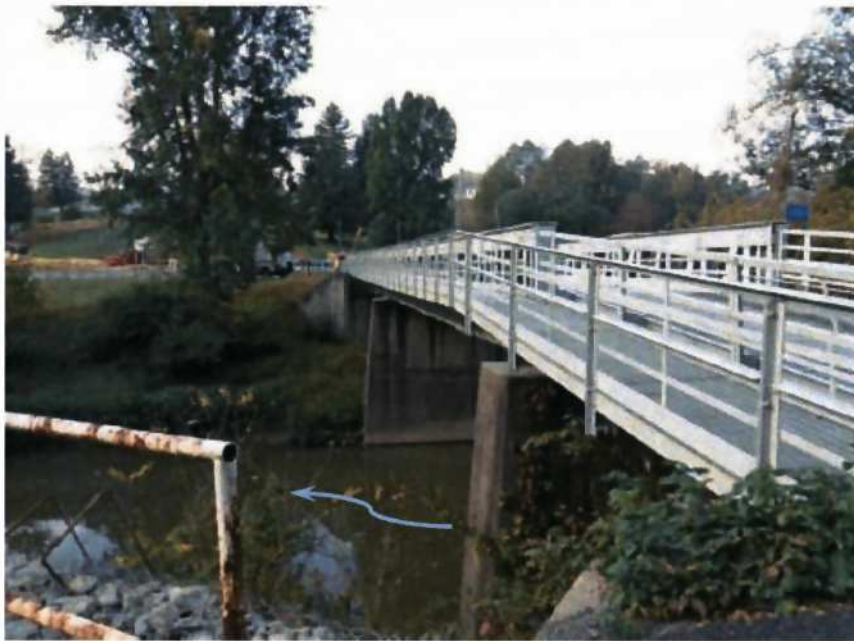
PHOTO 3 Existing bridge (downstream side).
