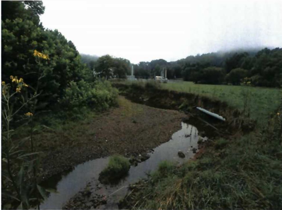
Streambank Stabilization Area – Looking East
