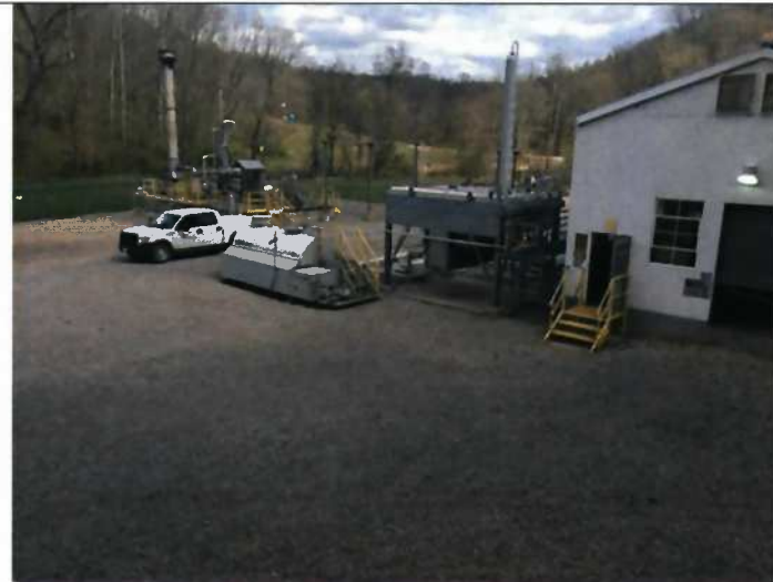
Photo: 4 Date: 4-28-2015 Comments: View of existing compressor building, and location of proposed new building, facing east.
