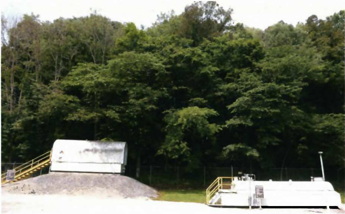
Photograph 3. Hillside beyond Station and Proposed Building Location
