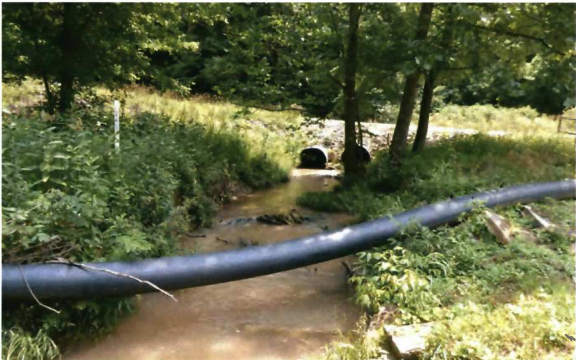
Photograph 4. Existing Culvert Crossing at Site Entrance (Looking Upstream)
