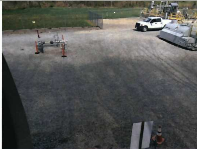
Photo: 3 Date: 4-28-2015 Comments: Overview of location of new compressor building, approximately 40 feet in front of the existing building, facing ENE.
