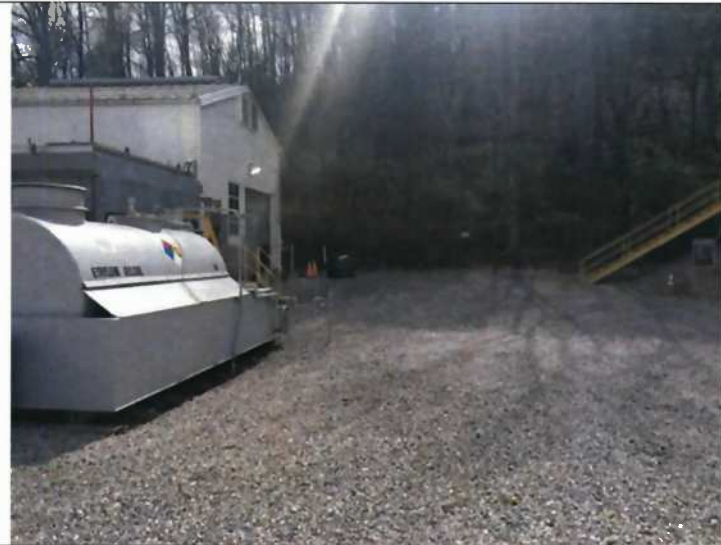
Photo: 2 Date: 4-28-2015 Comments: View of proposed workspace associated with the new building installation, facing WSW.
