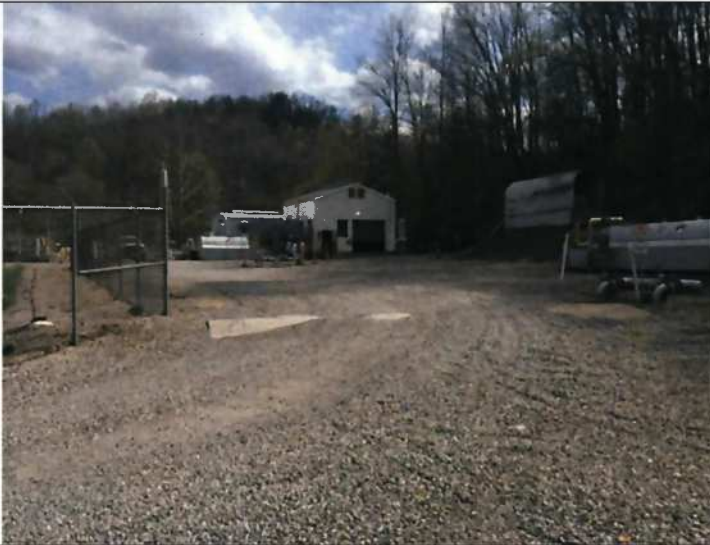
Photo: 1 Date: 4-28-2015 Comments: View of the existing gravel access drive and lot associated with the Maxwell Compressor Station, facing south.
