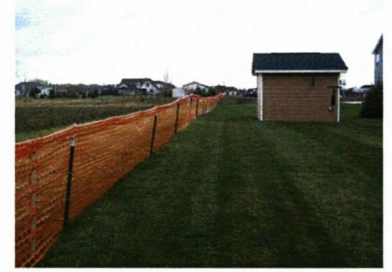
43A SUPPLEMENTAL 404 CWA BMP CONTROLS NTS DETAIL PROVIDED BY ANTERO MEDITERRAN LLC
