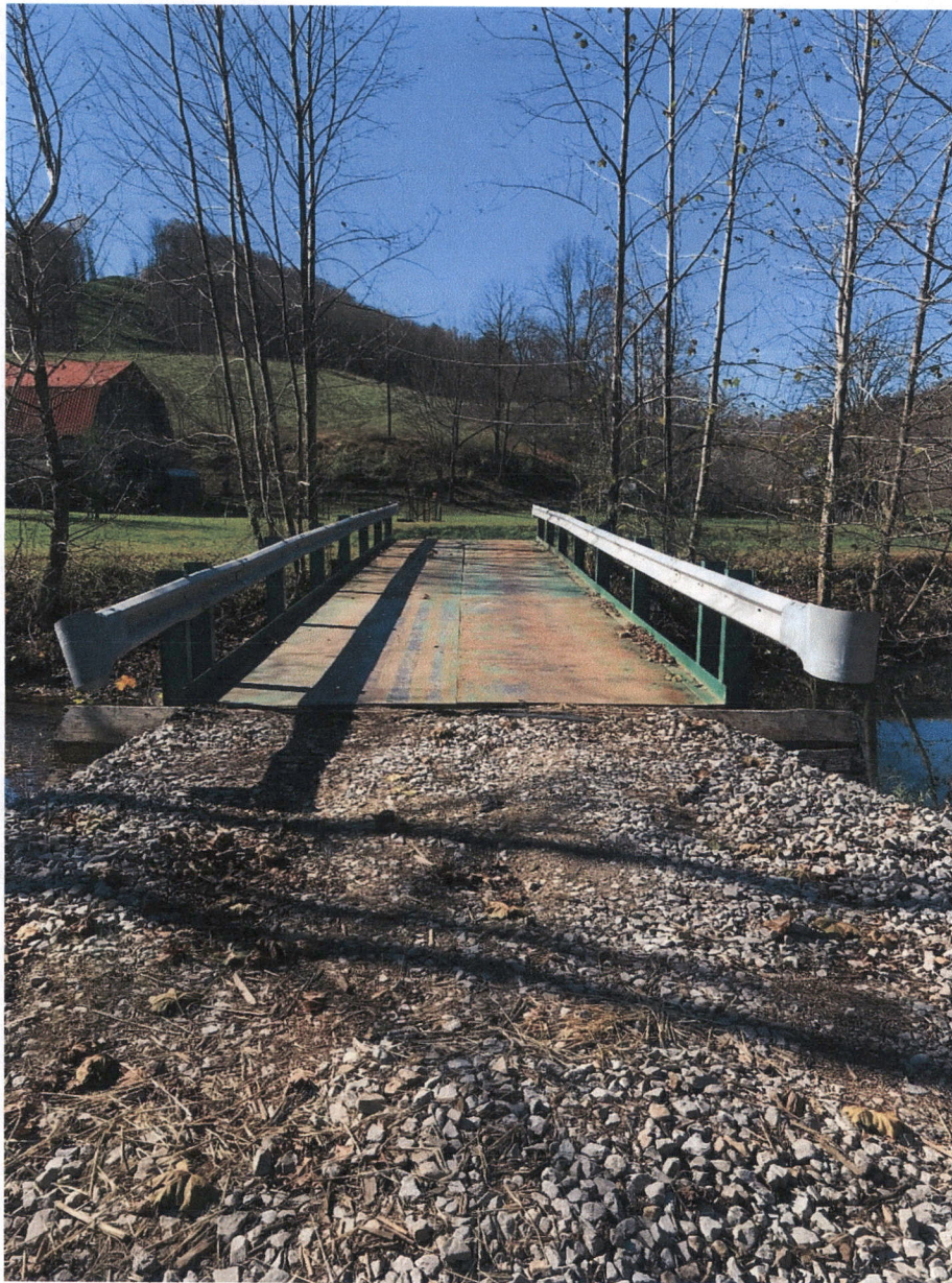
Figure 4: Current Bridge across McElroy Creek (Approach View)
