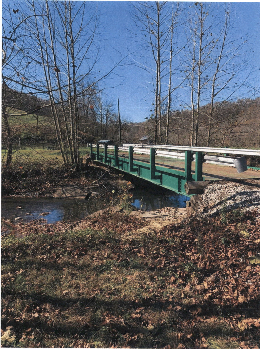
Figure 3: Current Bridge across McElroy Creek (Elevation View)
