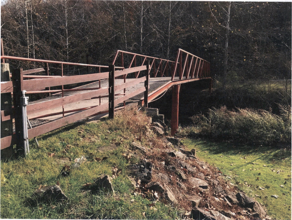
Figure 5: Upstream Existing Bridge across McElroy Creek
