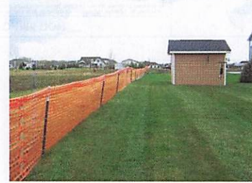
PHASE I: THIS IS ESSENTIALLY ORANGE SAFETY FENCE LIKE SHOWN ABOVE. THIS MEASURE IS PUT IN PLACE TO LET CONTRACTORS KNOW THAT NO WORK IS TAKE PLACE BEYOND THIS POINT. THIS CONTROL IS TYPICALLY UTILIZED WHEN THERE IS A WETLAND OR STREAM LOCATED IN THE AREA BUT NOT WITHIN APPROXIMATELY 100 FEET OF THE DISTURBANCE.
