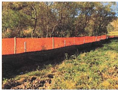
43 TEMPORARY SEDIMENT TRAP NTS
