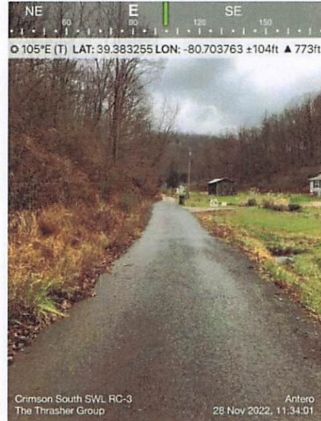
FACING SOUTHEAST SIGHT DISTANCE: 374'
