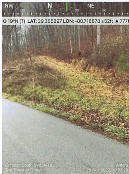
FACING NORTHEAST Looking at approach.
