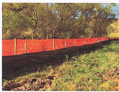
43 TEMPORARY SEDIMENT TRAP NTS
